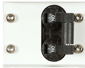
Circuit Breaker Closed (ON)
